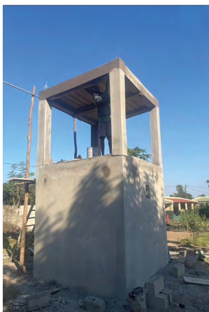
▲ Putting on the finishing touches – ready for the tank
