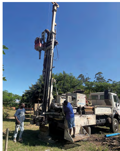
▲ Ready to drill the borehole
