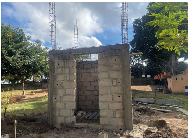
▲ The concrete beams being erected
