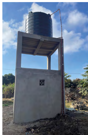
▲ The tank in place – just a bit further to go!
