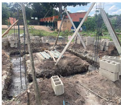
▲ Foundations for the water tower
