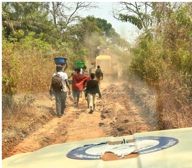
▲ Newly graded road
