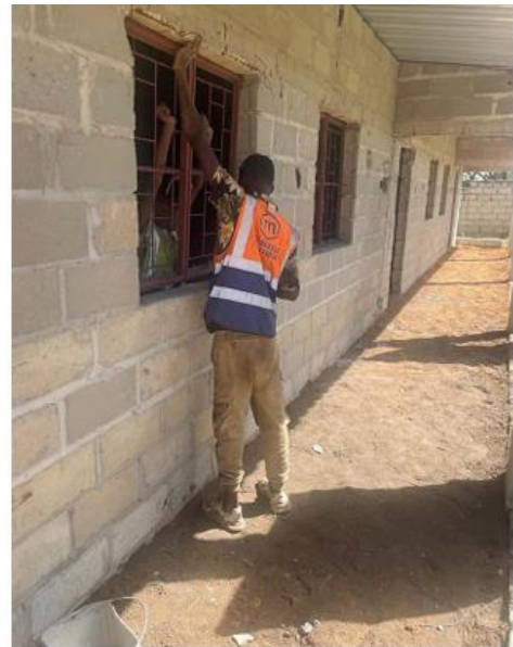
▲ Fitting the windows
