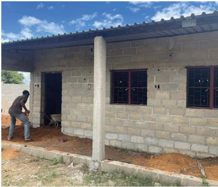
▲ The new classroom structure
