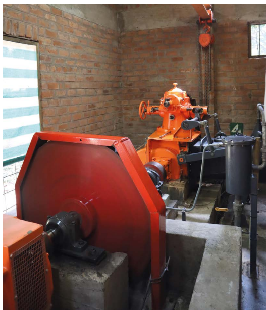
▲ The turbine at the hydro-electric plant
