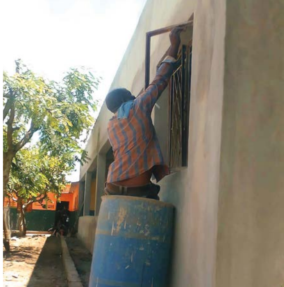
▲ Constructing the Canteen
