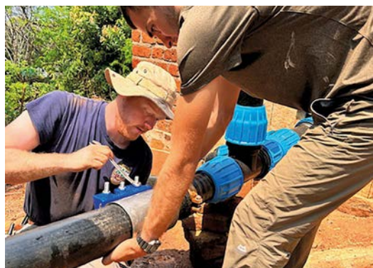
▲ Andrew and Isaac connecting pipes
