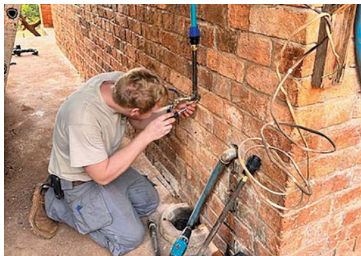
▲ At work on the plumbing
