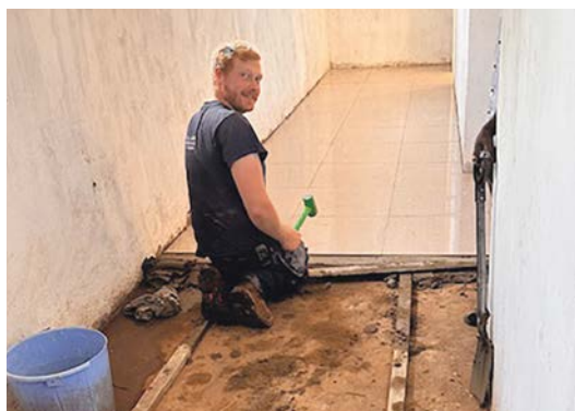
▲ Tiling the new hospital block
